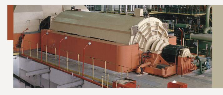
he liquid-cooled turbogenerators are well suited to central large power plants with power blocks of large output capacity. The requirements for a reliability and stable operation in the power grid of these generators are especially high.
